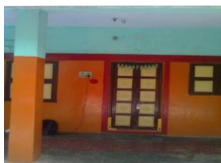
Figure.8. Short column effect. Unreinforced masonry infills placed up to partial height in frame panels adjoining the columns reduced column height. Such columns draw shear forces larger than designed
