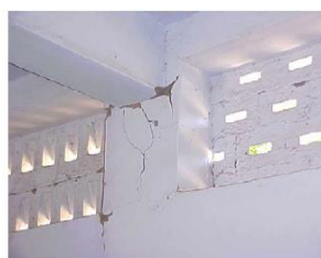
Figure.8. Short column effect. Unreinforced masonry infills placed up to partial height in frame panels adjoining the columns reduced column height. Such columns draw shear forces larger than designed
