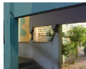
Figure.8. Short column effect. Unreinforced masonry infills placed up to partial height in frame panels adjoining the columns reduced column height. Such columns draw shear forces larger than designed
