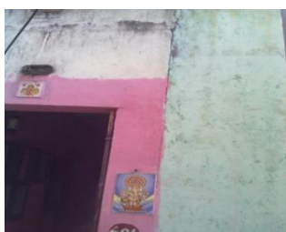
Figure.9. In some areas, like this part of row constructions are common, with little or no space left between adjoining buildings. At the interface between such buildings, infills are sometimes made only in one of the two buildings. There were no infills in the upper stories of the building on the left. The building on the right suffered a ground storey
